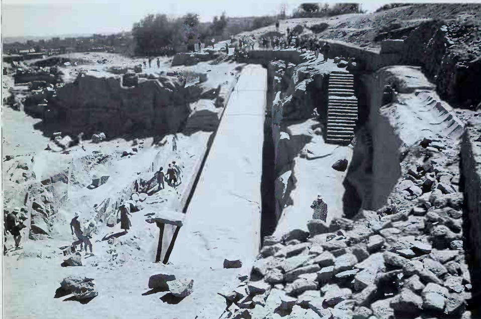
The unfinished obelisk at Aswan, probably dating to the 18th Dynasty. If the discovery of a major geological flaw had not halted work on it, this would have been the largest obelisk ever quarried.
