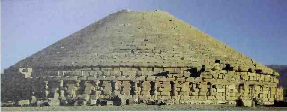
A circular mausoleum at Le Medracen, near Batna in Algeria, c. 200/150 BC. The roof is in the form of a stepped pyramid, and the vertical face is ornamented with Doric half-columns.
